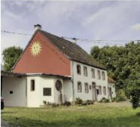
The house purchased in Germany in Lierfeld
